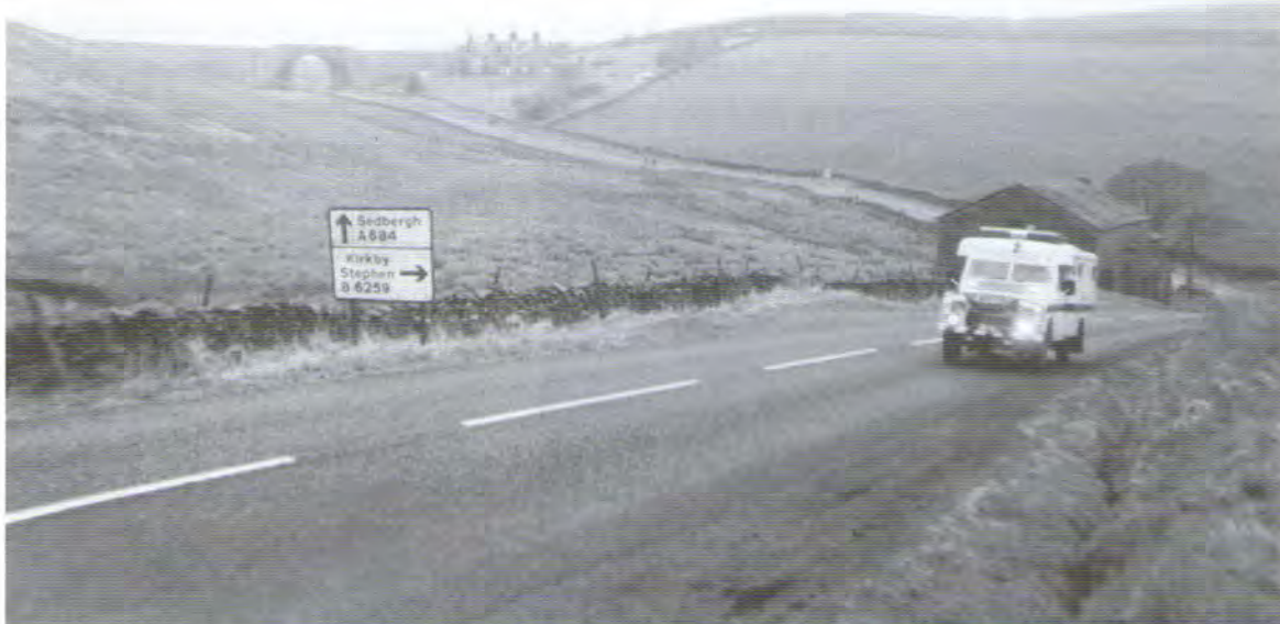
Settle - Carlisle Bridge, Garsdale
