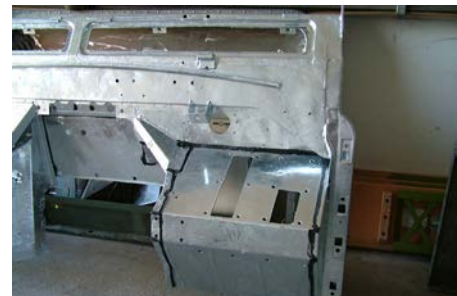
Above: Bulkhead fixed!
