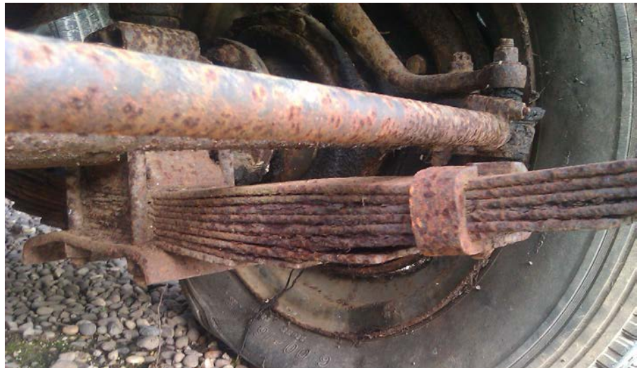
Above: A heavily corroded spring
