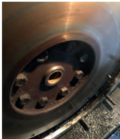
New bush fitted after old one gently cut out
